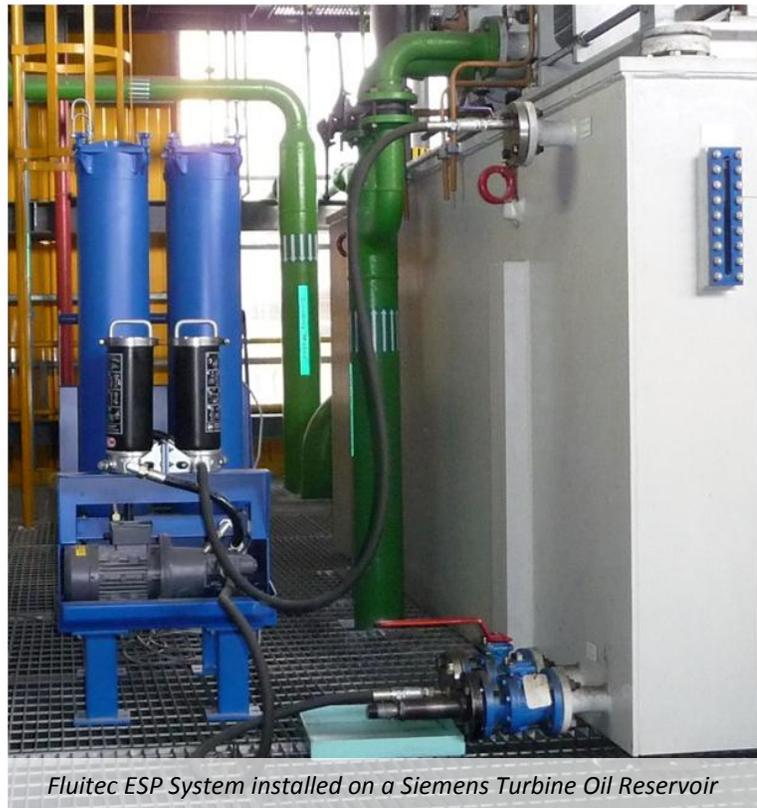
*Fluitec ESP System installed on a Siemens Turbine Oil Reservoir*
